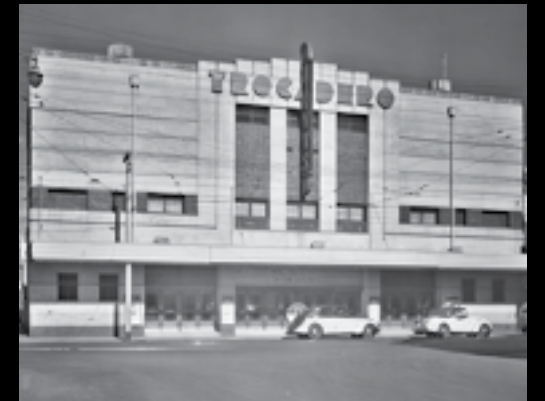
Trocadero Theatre, Hopkins Street, Footscray 1941
