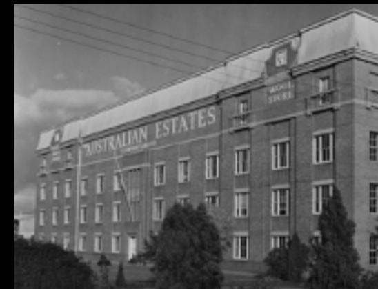
Australian Estates Woolstore Sunshine Road West Footscray. 1950
